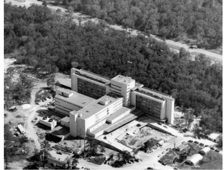
Construction of MD Anderson in 1952
